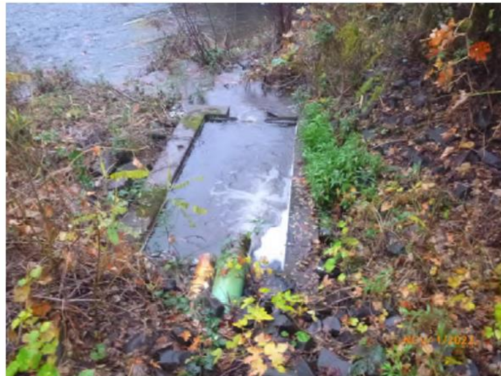
Photo showing collected seepage through dam of 150 gallons per minute +/-
