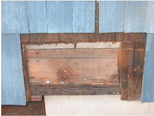
Figure 5 – The original white-painted clapboards can be seen behind several layers of modern shingles
