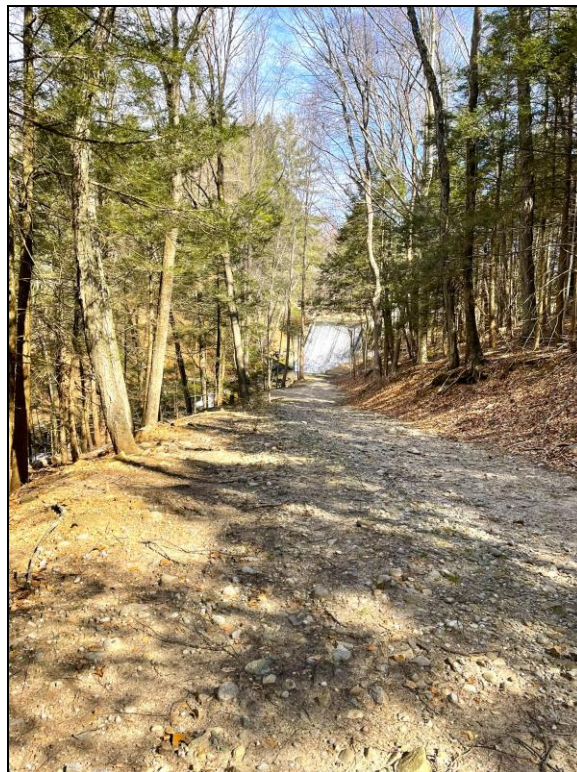
Photo 10. View of Great Hill Reservoir dam.
