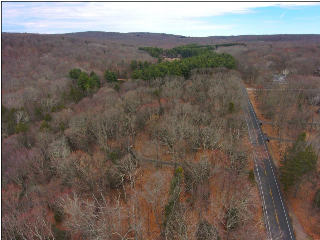
Photo 1. Drone view of SE-5 access road from Squantuck Rd looking north.
