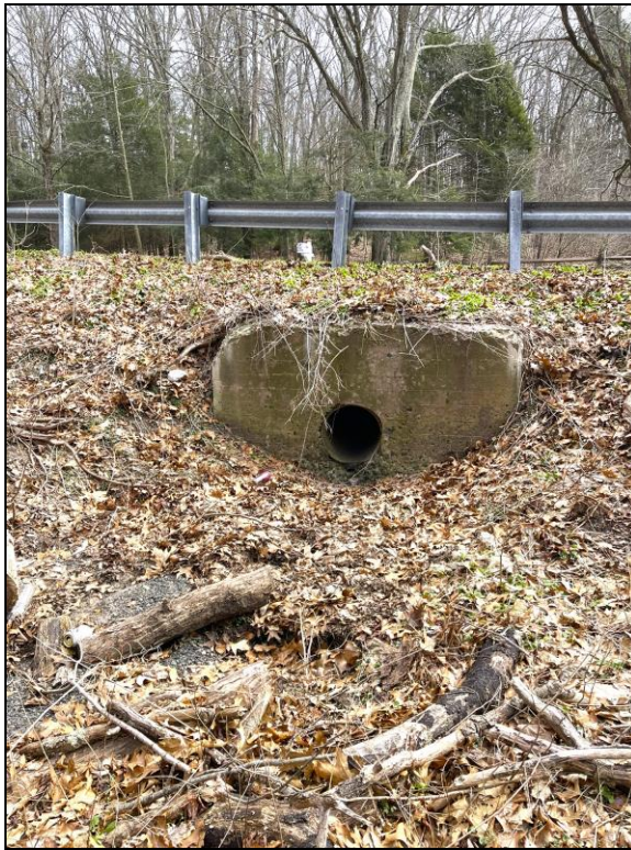
Photo 7. Headwall for Squantuck Road stormwater discharge looking east.
