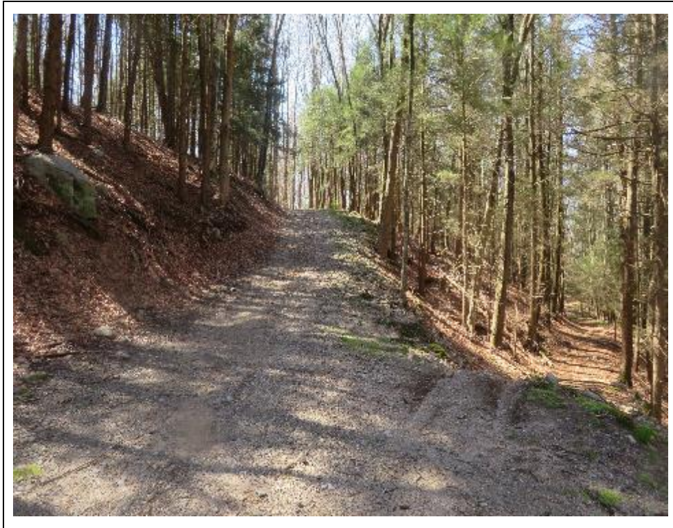
View east along accessway roadway (Photo7)
