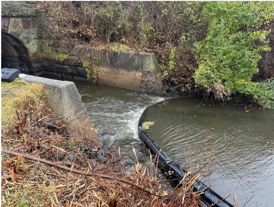
Figure 7: Documented backflow. Water on the right is from Furnace Pond. A visible imbalance is present and highly organic water is entering Lake Saltonstall.
