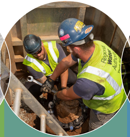
Our Water Mains & Service and Construction crews perform a lot of complex work every day on our more than 1,700 miles of pipeline to improve water service reliability. Anthony Spero (left) and Anthony Dellacamera , both Construction Utility Techs , work on a gate valve in North Haven. Projects like this avoid service disruptions and reduce water waste caused by leaks.
